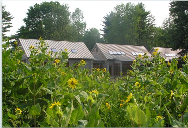
sunflowers growing in the dosing field (wastewater treatment)
