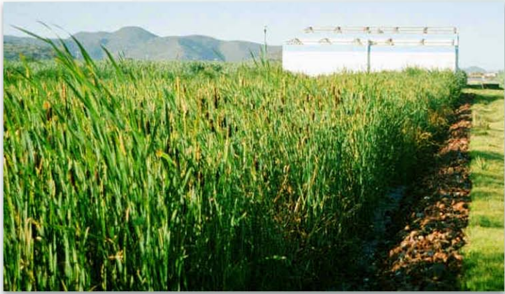
constructed wetlands (foreground) with trickling filters (background)
