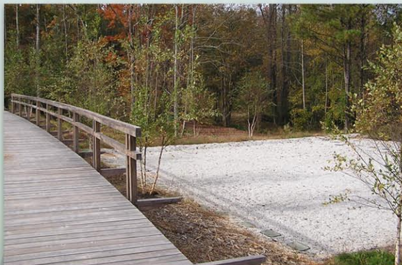
recirculating sand filter
